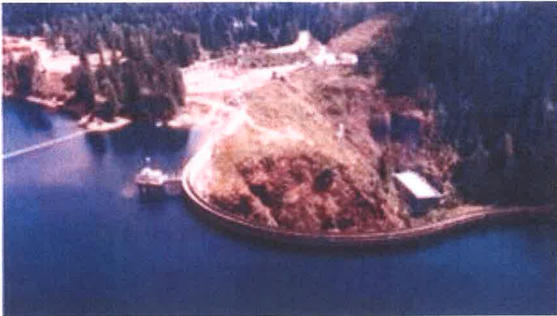
Figure 2.6 – Cushman No. 1 Dam
