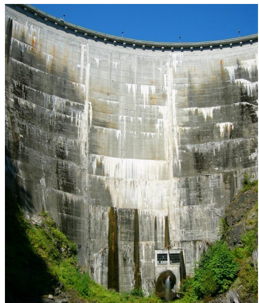
Cushman No. 1 Dam
