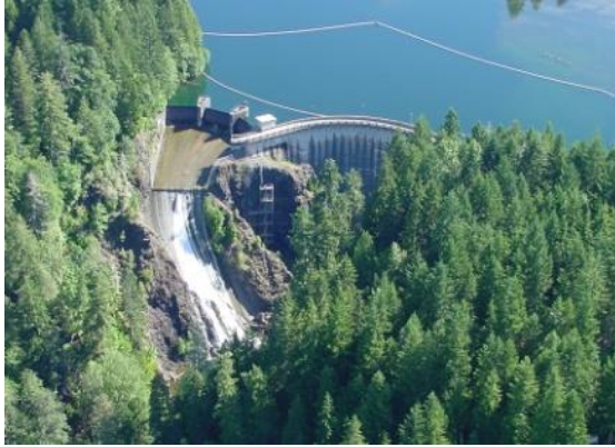
Cushman No. 2 Dam
