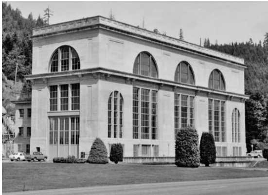
Cushman No. 2 Powerhouse
