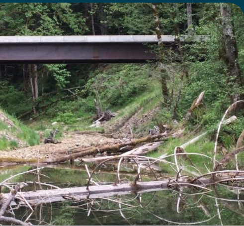
▲ Bridges protect the environment and provide safe transport.
