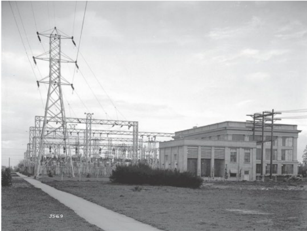
Cushman & Adams Substations – April, 1937
