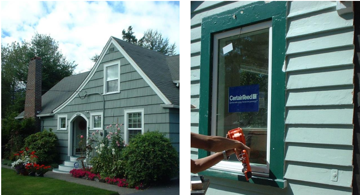
Figure 6-1 Residential Home Weatherization (courtesy of Tacoma Power)
