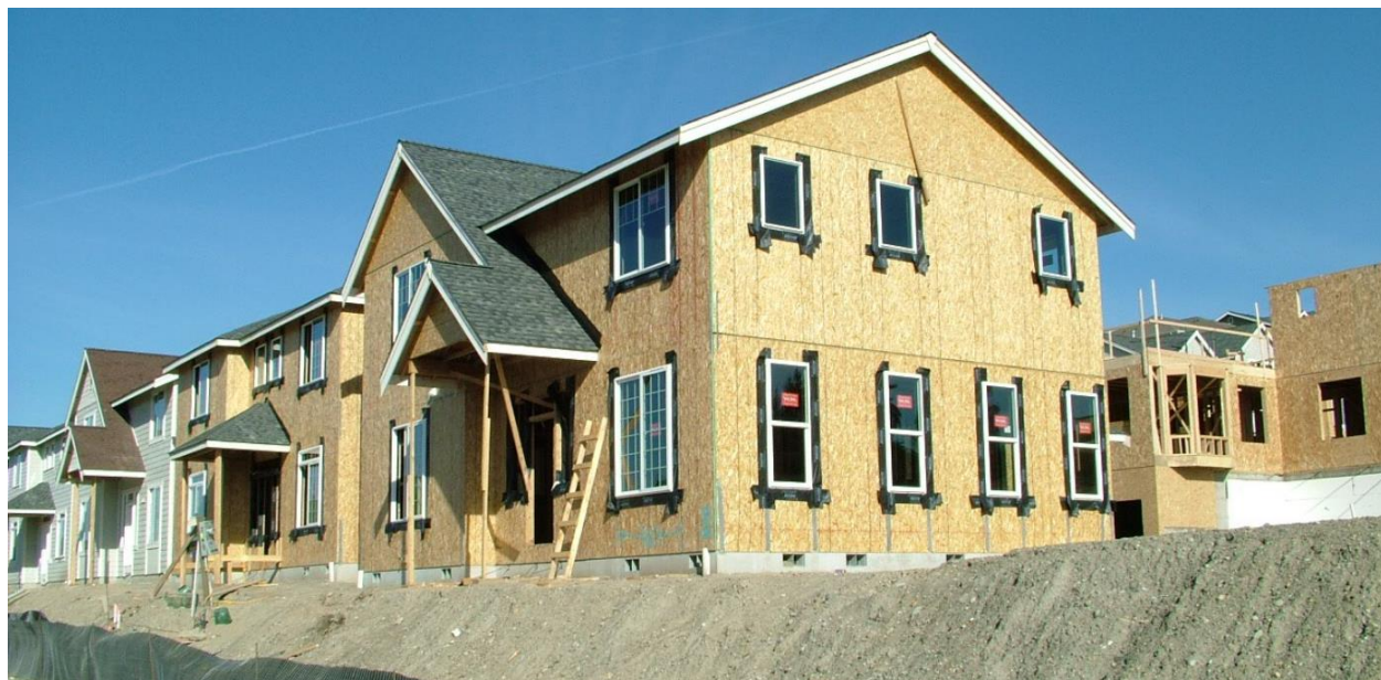
Figure 4-3 Townhomes Under Construction (courtesy of Tacoma Power)
