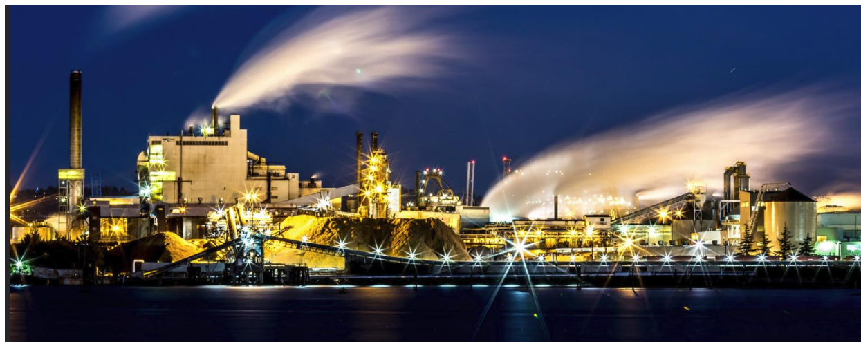
Figure 6-19 WestRock Pulp Mill (courtesy of Rob Green)
