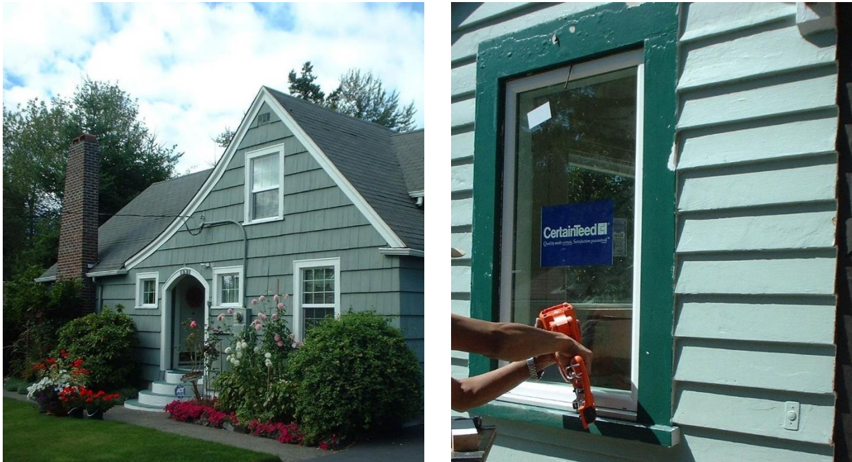
Figure 6-1 Residential Home Weatherization (courtesy of Tacoma Power)
