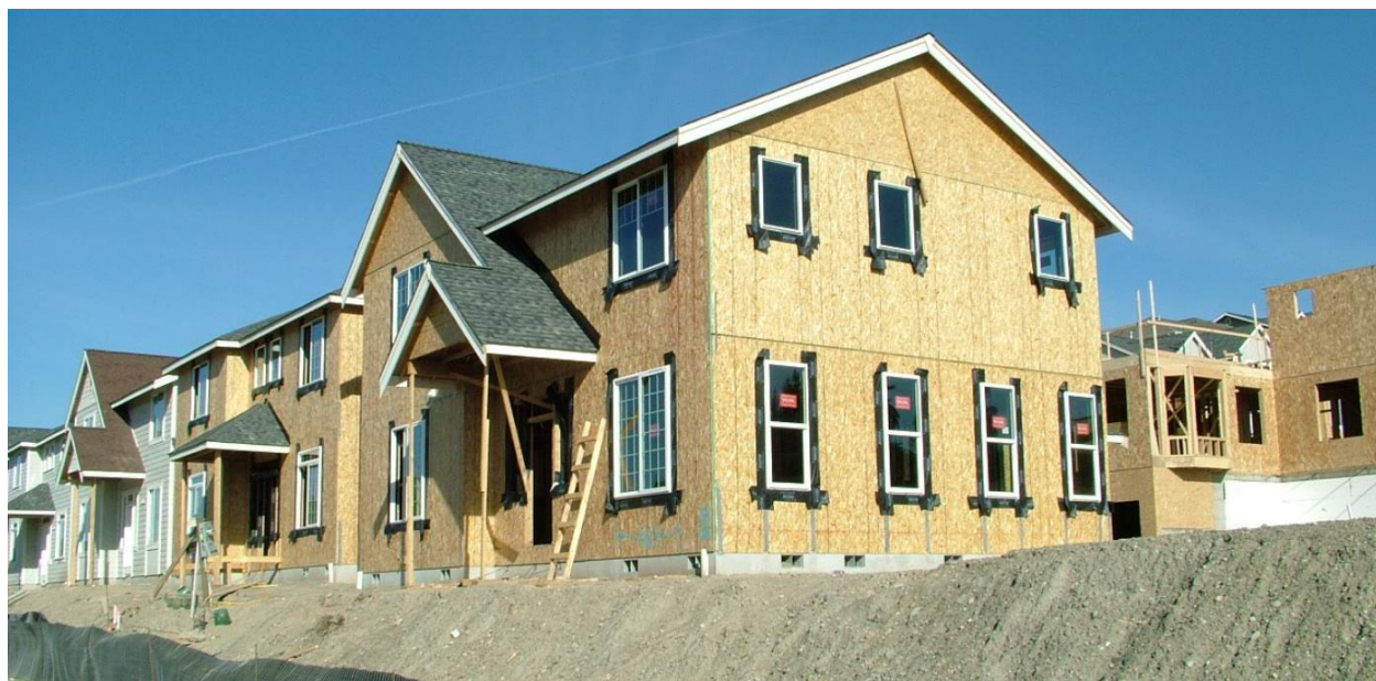
Figure 4-3 Townhomes Under Construction (courtesy of Tacoma Power)
